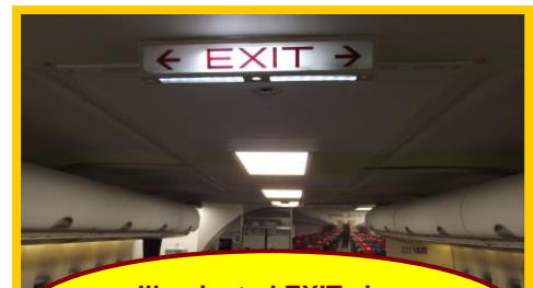
Illuminated EXIT sign controlled by the FAP
